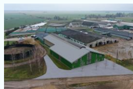
Diary Farm modernization project
